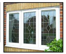
To create equal glass areas within the window design, it is necessary to introduce 'dummy sashes'.
